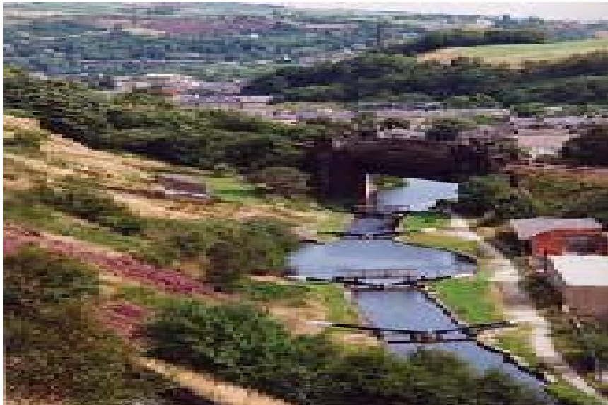
The Railway Bridge at Gauxholme.
